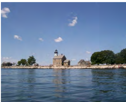
Lighthouse at Sheffield Island
