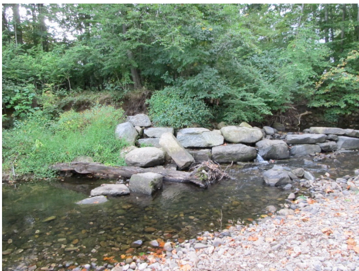
Remaining pieces of J-hooks that were installed in early 2000s at site SM5. Stream bank erosion can be seen in the background.
